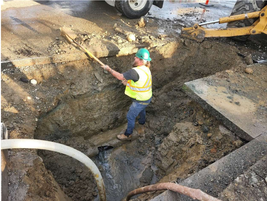
IMAGE | MOORLAND LEAK REPAIR
