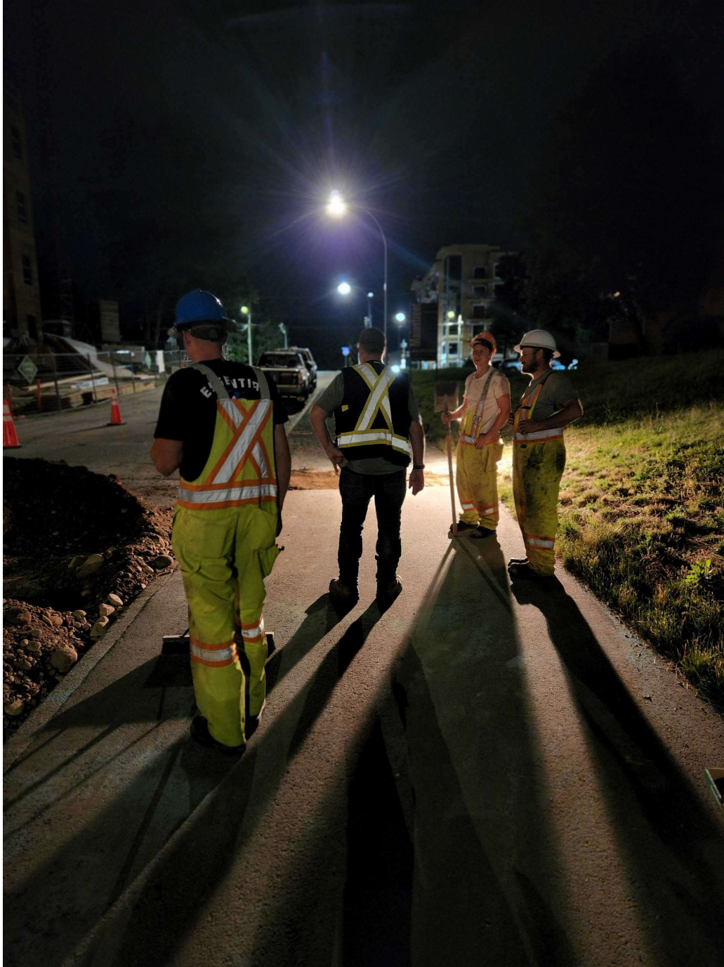
IMAGE | MIDNIGHT EMERGENCY TIE-IN – TIMS STREET
