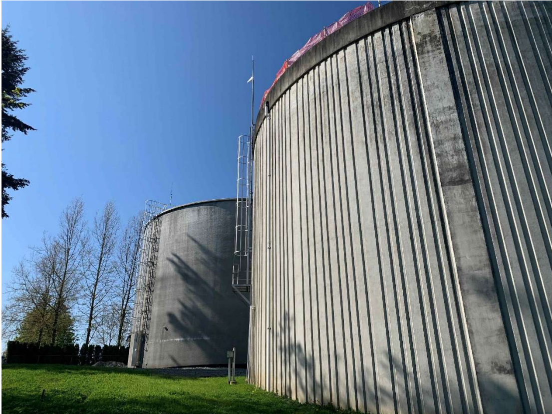
IMAGE | RESERVOIR B (left) and RESERVOIR C (RIGHT).
