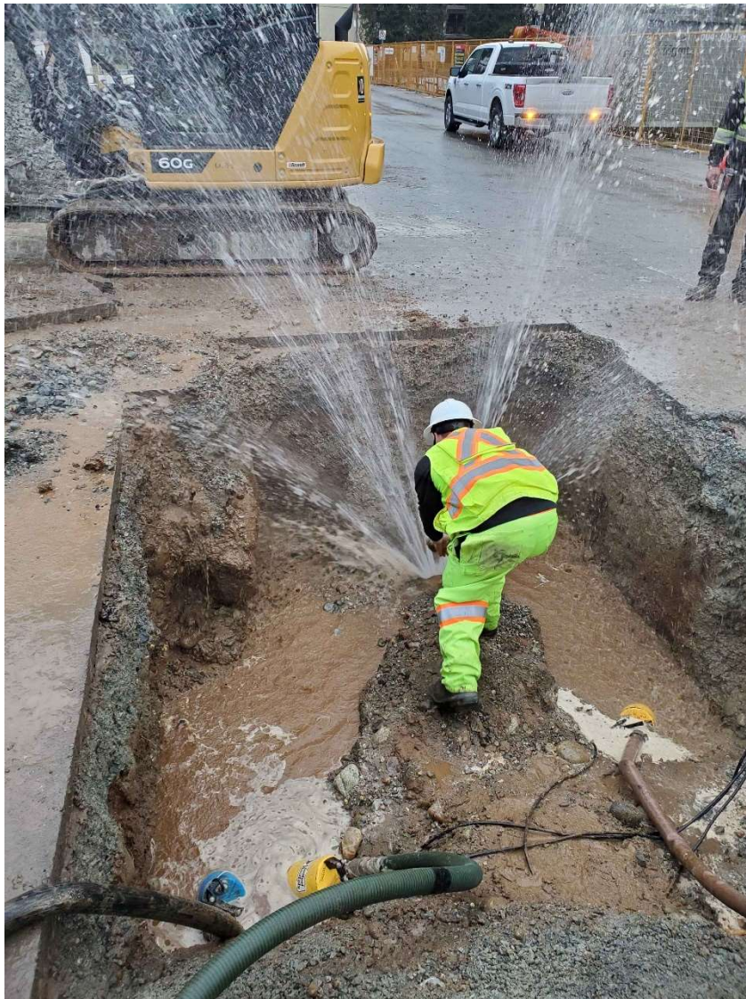
IMAGE | TIMS STREET LEAK REPAIR
