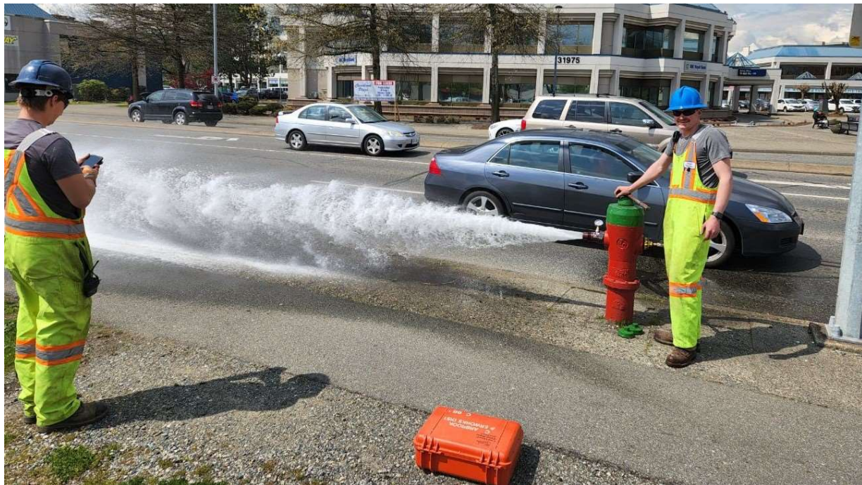
IMAGE | WATER SYSTEM FLUSHING IN PROGRESS.
